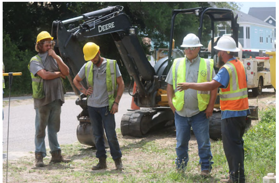
Resident confronts illegal gas pipeline installation
