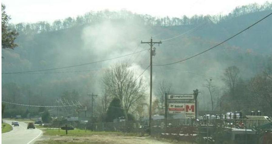
Figure 3. Operating Asphalt Plant
