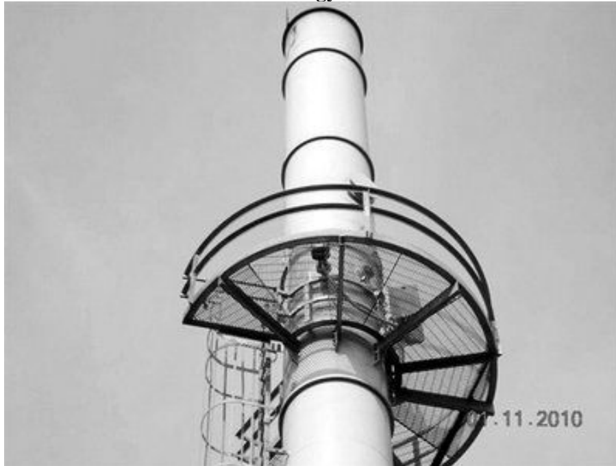
Smokestack of a Waste to Energy Biomass Gasification Plant 1
